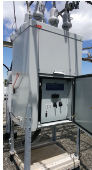
Pictured: 15 kv circuit breaker
