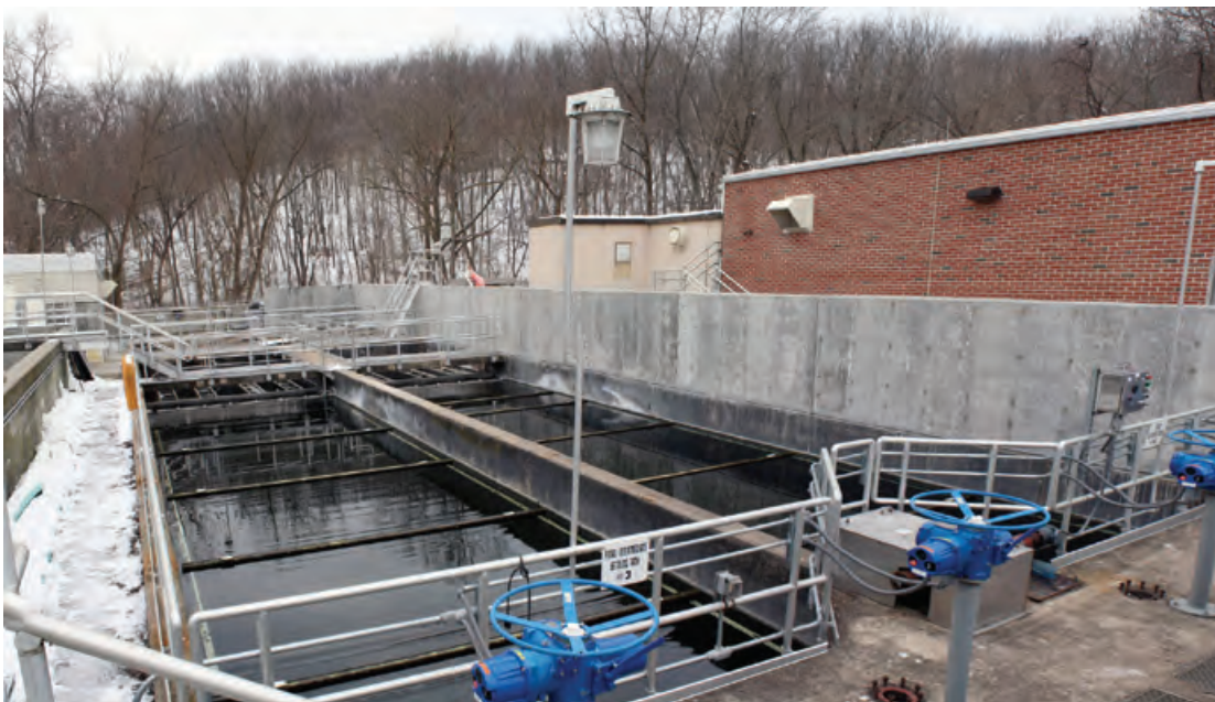
G FINAL SETTLING TANKS
